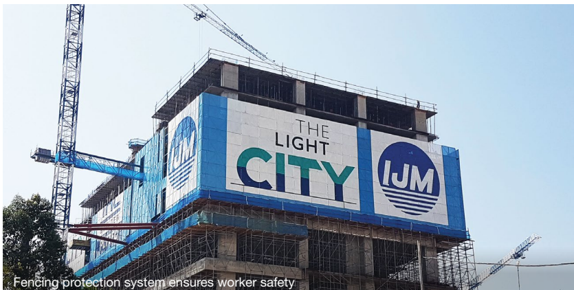
Fencing protection system ensures worker safety
