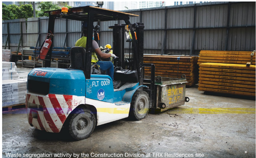
Waste segregation activity by the Construction Division at TRX Residences site
