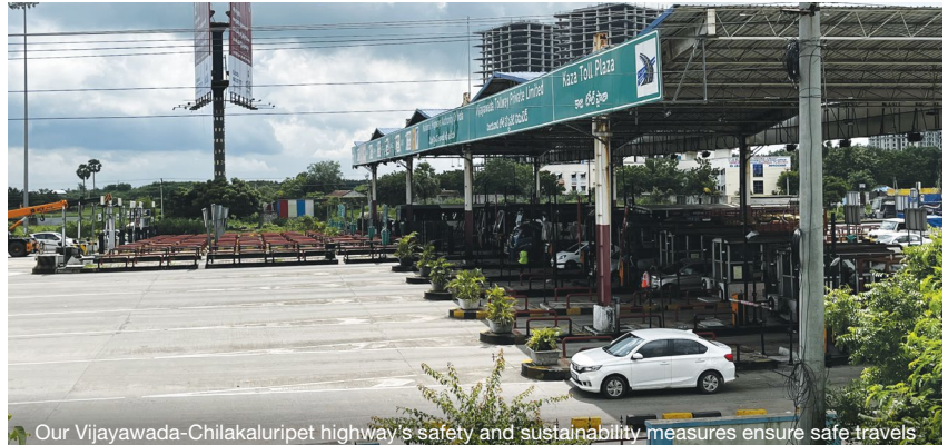
Our Vijayawada-Chilakaluripet highway's safety and sustainability measures ensure safe travels
