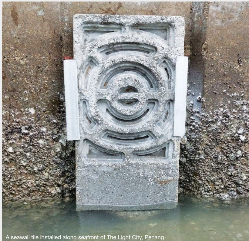
A seawall tile installed along seafront of The Light City, Penang
