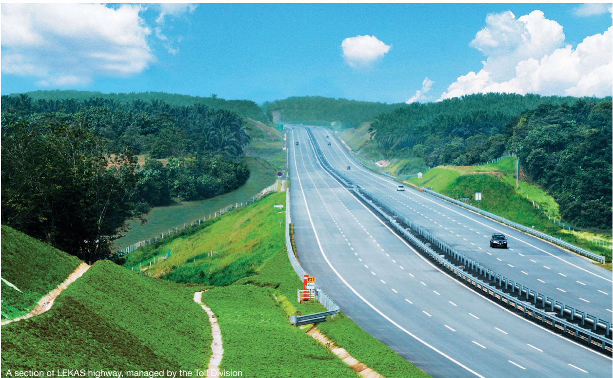
A section of LEKAS highway, managed by the Toll Division
